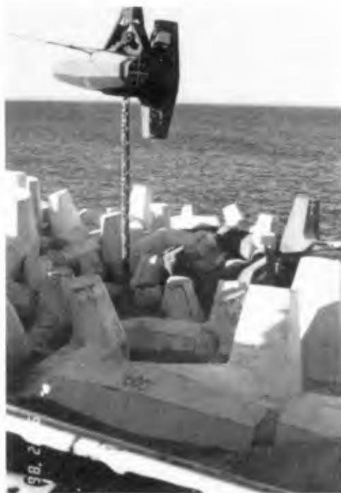
Figure 2: Instrumented Dolos and Chain Assembly
