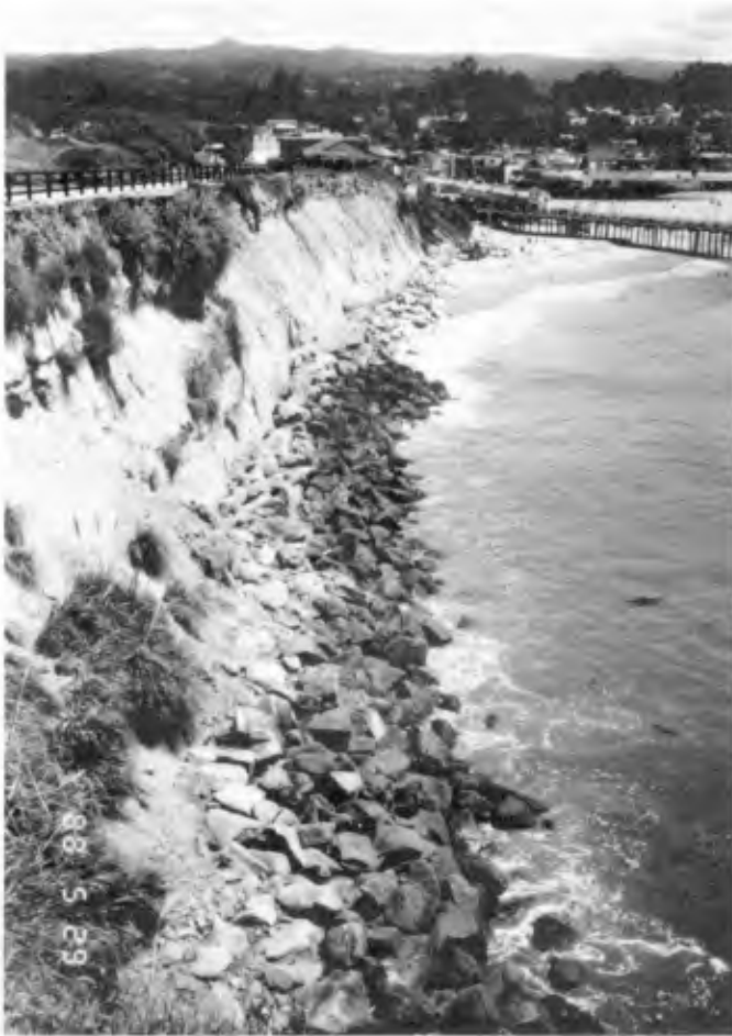
Figure 9 - Seawall near Capitola (May 1988)
