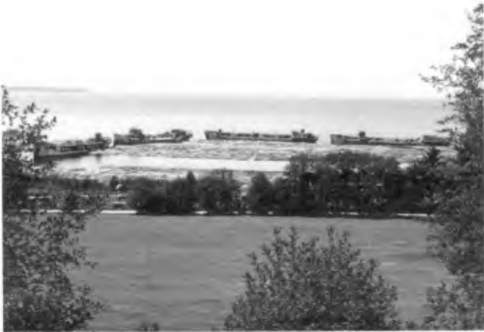
Fig. 5. The floating breakwater at Powell River, comprised of ship hulls.
