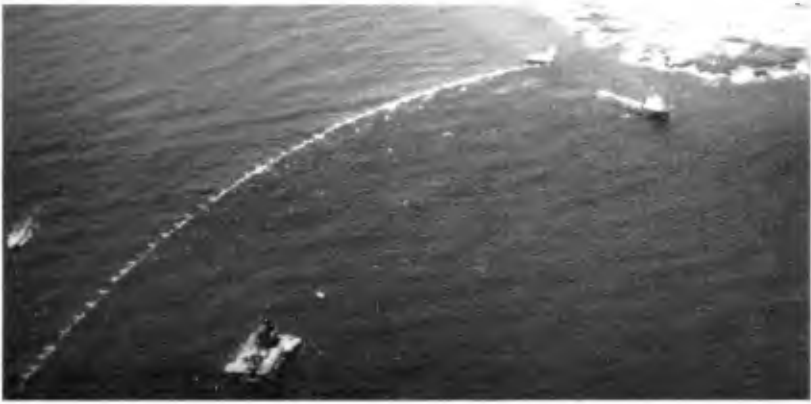
Figure 10. Aligning Pipe Section 1, Keahole Point
