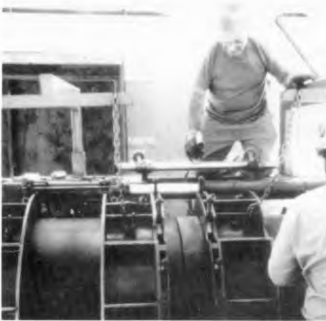
Figure 4. Polyethylene Pipe Thermal Butt Welding
