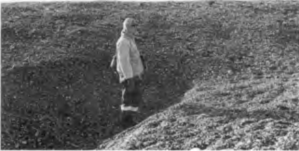
Fig. 8. A seepage hollow formed on the landward side of Hurst Beach on 23 November 1984. Note the angle of repose slope. The man is 1.80m tall.
