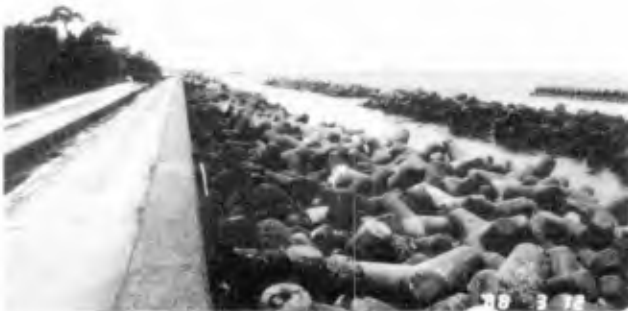
Photo 7. Left-hand side view of the experimental works.
