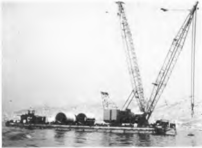
PIPE LAYING BARGE
