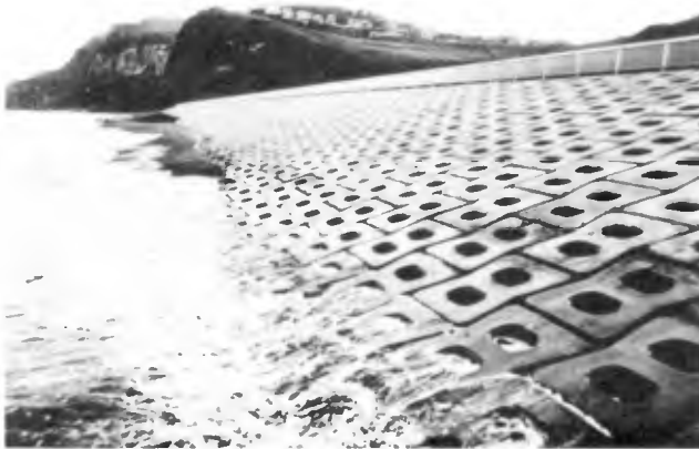
Photo 1. Experimental seawall immediately after the completion (1982).
