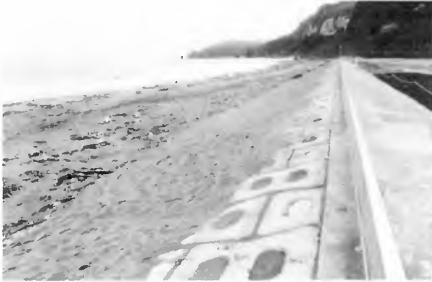
Photo 2. A later view of the experimental seawall.
